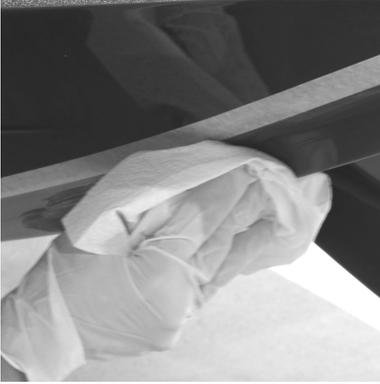
Thoroughly clean the area with isopropyl alcohol using paper towels or a clean rag. Repeat until there is no sign of residue. **Do not** use paint thinner or other petroleum based cleaners as they will compromise the bond of the adhesive. Always remember to wear protective gloves.
