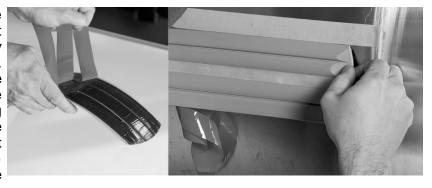
Once fully attached, use the burnishing tool to apply additional pressure to the entire PontoonGuard, ensuring the pressure sensitive adhesive is firmly attached.
