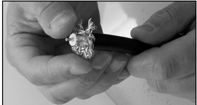
Figure 87: Flaring the Braid
