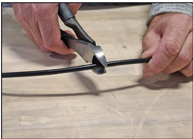
Figure 59: Cutting the Cable
