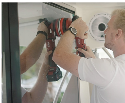
Image 6.2: Buffing glass surface with G200 glass polish.
