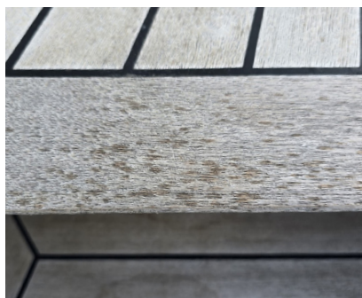
Image 4.2: Mold/mildew spots on a teak deck with heavy graying.
